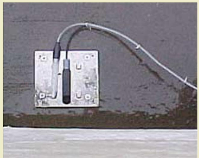
Figure 22 – AV sensor and strainer mounted to a plate at the bottom of a storm channel
