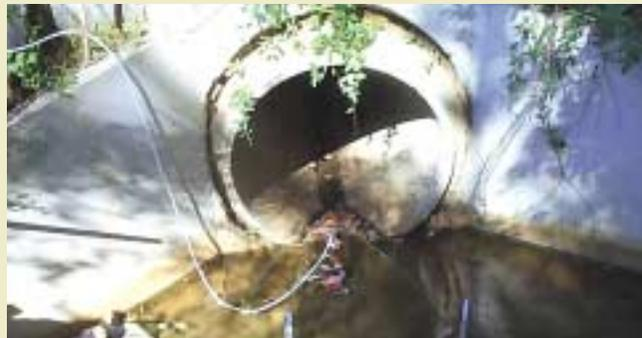
*Figure 10 – Sampler intake in storm pipe*
