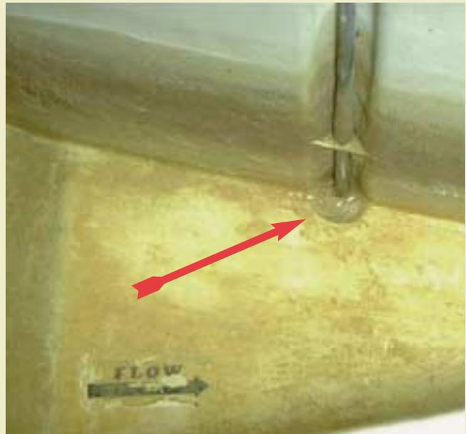
Figure 20 – Close-up of bubbler hose end
