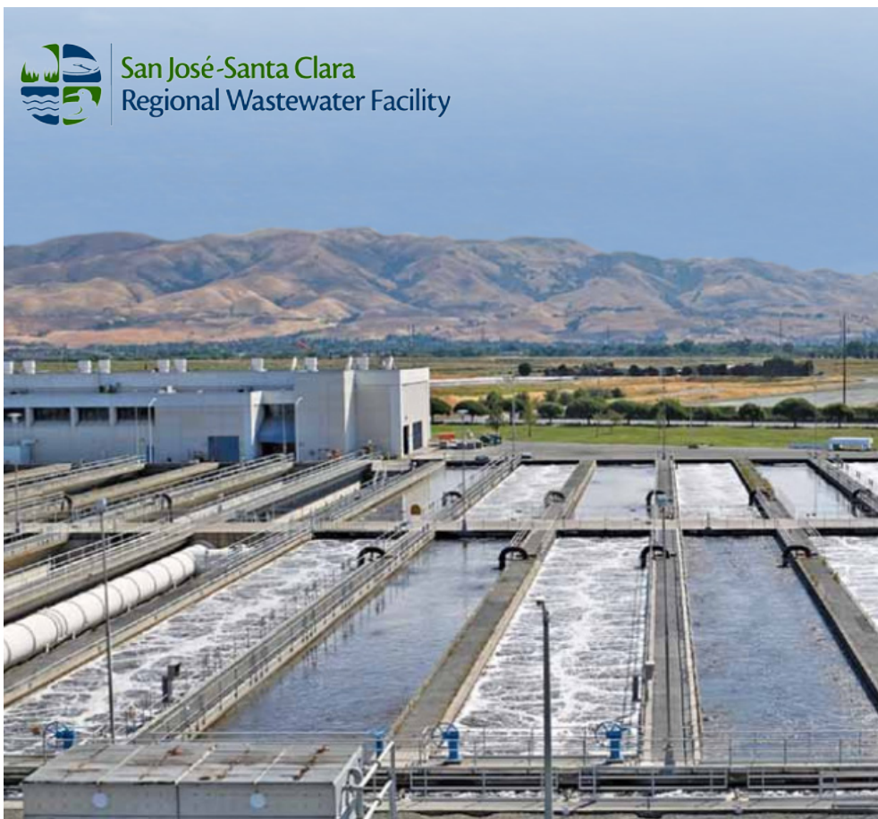
San Jose/Santa Clara Regional Wastewater Plant
